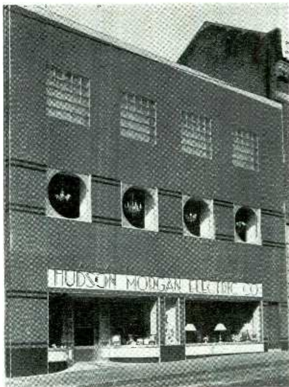
EXTERIOR — The new and the old present a striking contrast.
